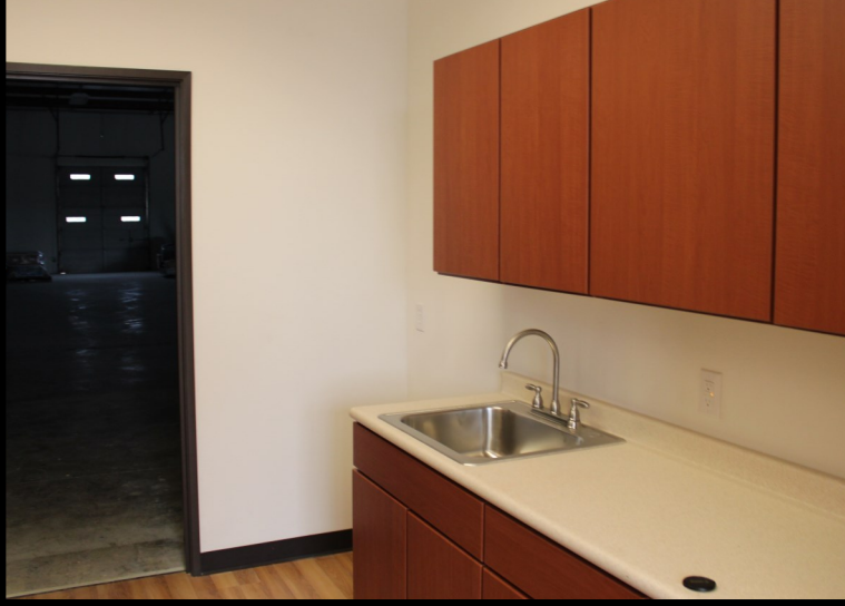
Kitchenette in built out offices in Suite H
